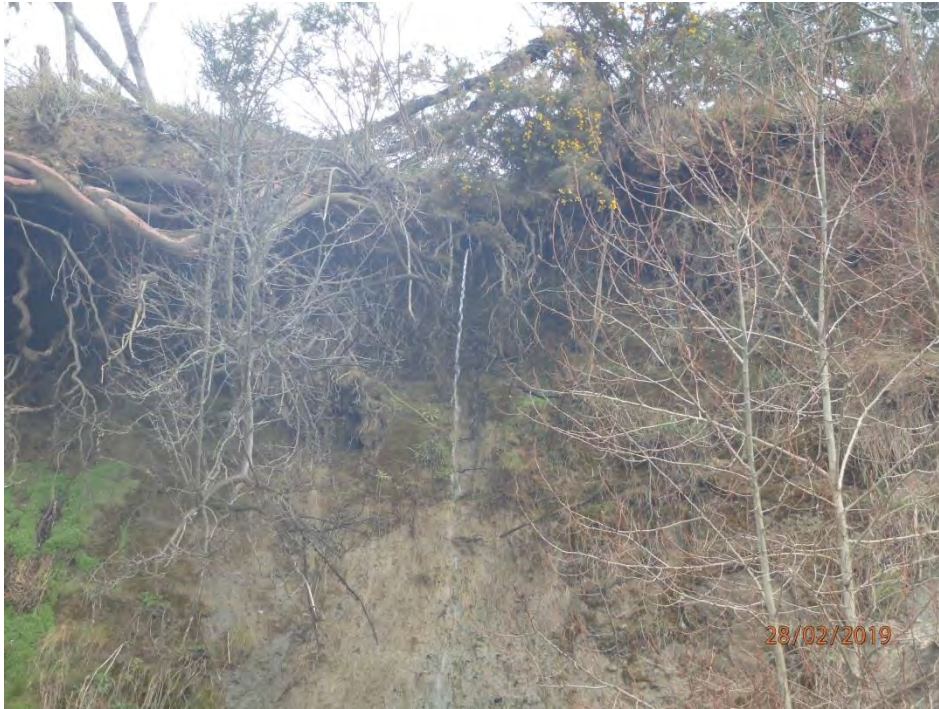
DRAINAGE OUTFALL PIPE LOCATED IN THE BACKSHORE ZONE ADJACENT TO BEACH UNIT 11.
