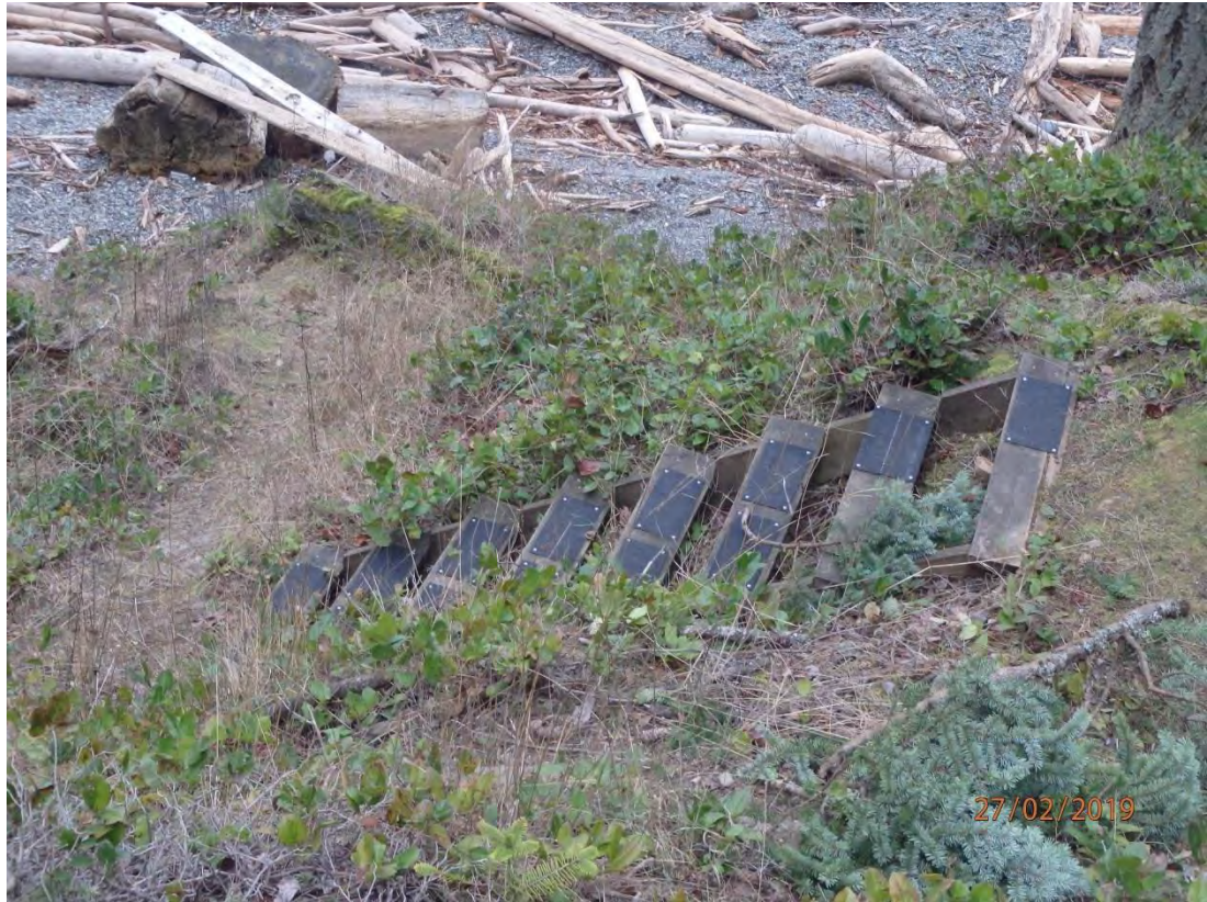
STAIRWAY ACCESS IN THE BACKSHORE ZONE - BEACH UNIT 26.
