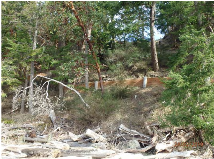
LOOKING EAST TOWARDS A WOODEN RETAINING STRUCTURE FORMING PART OF A BEACH ACCESS TRAIL IN BEACH UNIT 4. NOTE MINIMAL FOOTPRINT AND RETENTION OF VEGETATION.
