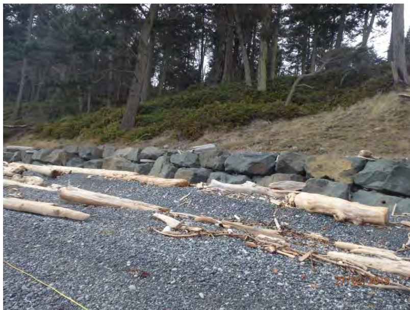
LOOKING WEST TOWARDS THE RIP-RAP RETAINING WALL LOCATED IN BEACH UNIT 24.
