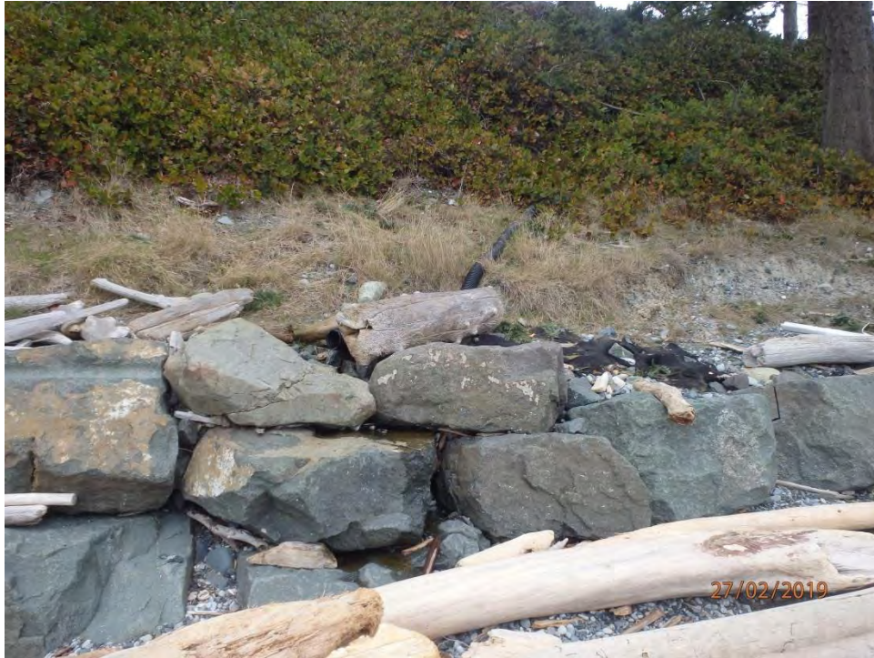
RIP RAP RETAINING STRUCTURE AND OUTFALL PIPE - BEACH UNIT 24.
