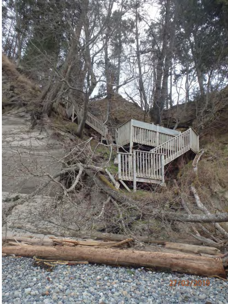
STAIRWAY ACCESS IN THE BACKSHORE ZONE - BEACH UNIT 29.
