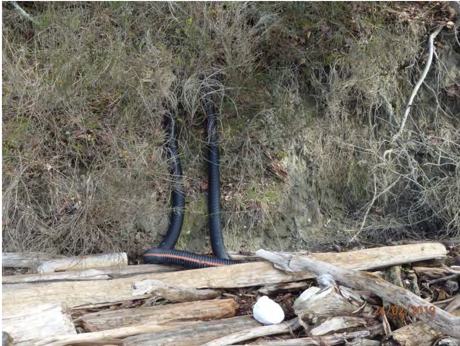
STORM OUTFALL PIPES DISCHARGING ONTO THE BEACH - BEACH UNIT 4.
