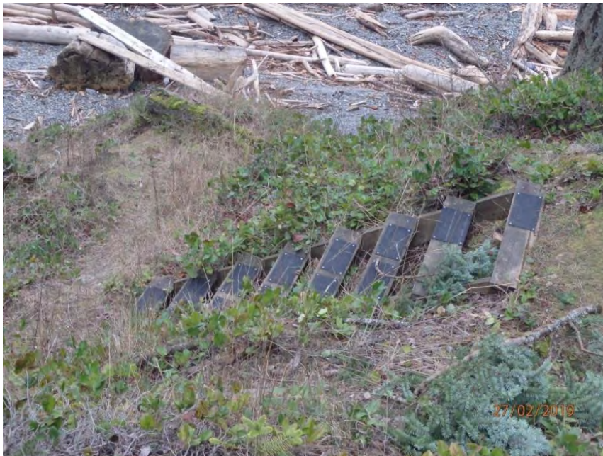
MINIMAL BEACH ACCESS STAIRWAY ASSOCIATED WITH BEACH UNIT 26.
