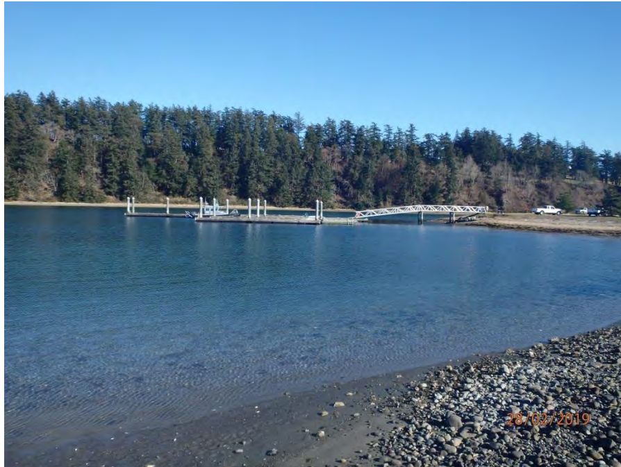
LOOKING EAST OVER THE LAGOON TOWARDS THE MARINA THAT REPRESENTS THE MAIN ACCESS POINT FOR JAMES ISLAND.
