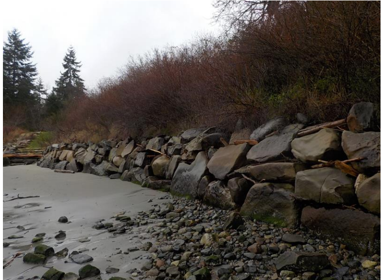
Riprap armouring on foreshore Crown land and suitable spawning habitat. Evidence of wave scouring at hard armouring with exposure of cobble layer below spawning sediment. Galiano Island Photo: RC de Graaf
